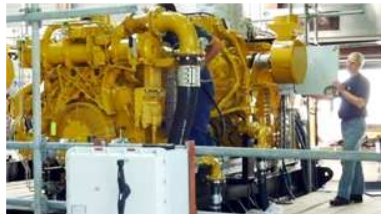
1.5 MW biogas engine generator set 53
