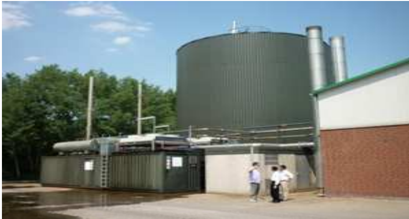
Biogas plant generating 1 MW of electricity and 1 MW of heat plus organic fertilizer
